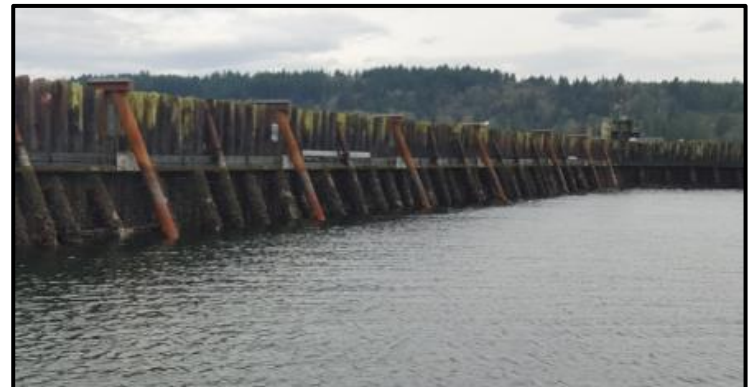
EXISTING CREOSOTE TIMBER PILE BREAKWATER
